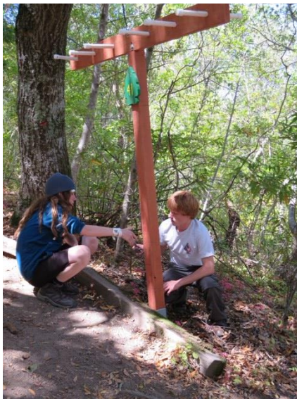
Checking vertical alignment.
