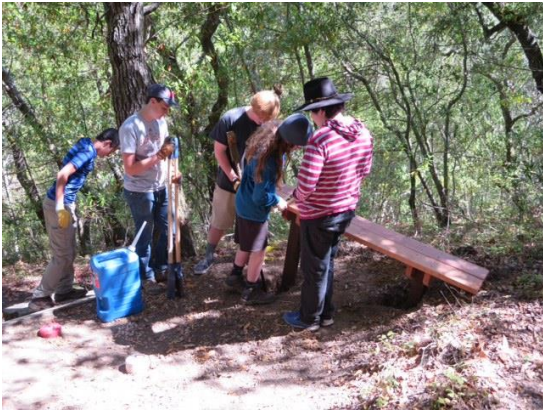
Setting the height on a new bench.
